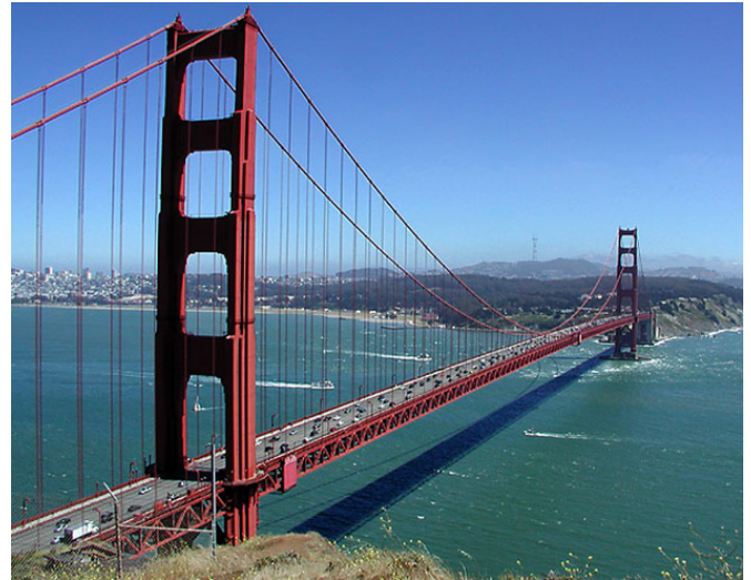
The Golden Gate Bridge looking south toward San Francisco
