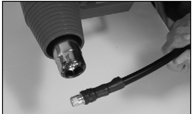
Figure 63: Applying the Heat Shrink Tubing
