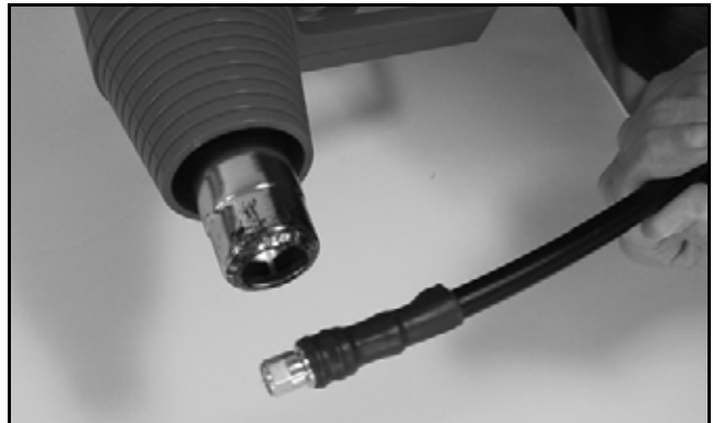
Figure 63: Applying the Heat Shrink Tubing
