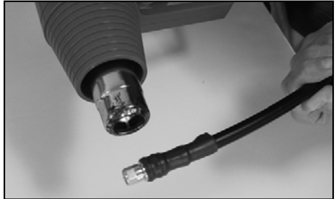
Figure 65: Applying the Heat Shrink Tubing
